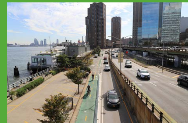
This on-street path along the East River forms a piece of the Manhattan Waterfront Greenway.
