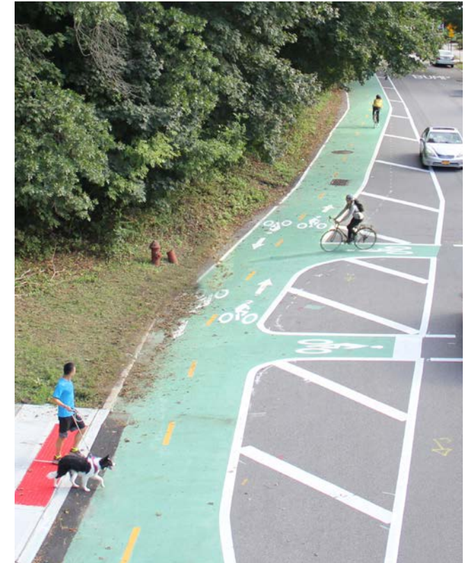
▲ This on-street path along 230th St in Queens provides access to Alley Pond Park and the Eastern Queens Greenway
