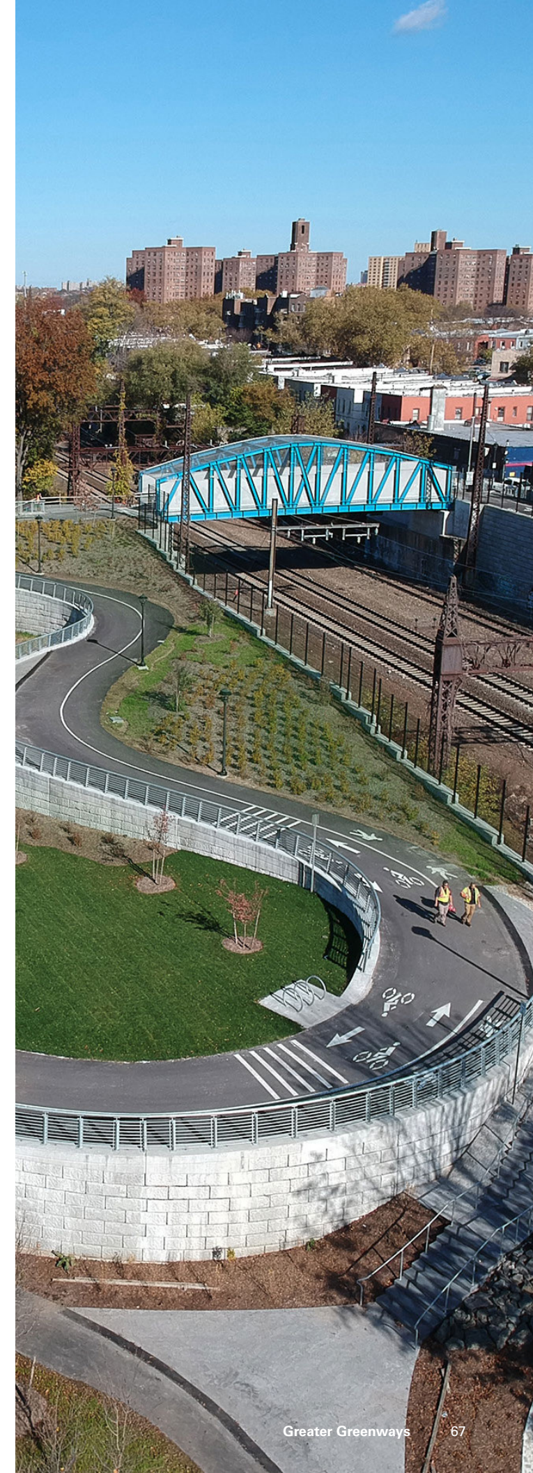
This segment of the Bronx River Greenway in Starlight Park weaves along the river and over Amtrak tracks, integrating seamlessly with the adjacent neighborhoods.
