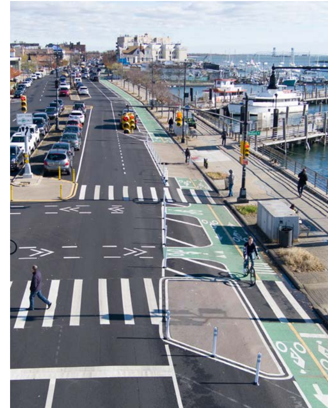
▲ A segment of the Brooklyn Waterfront Greenway along Emmons Ave in Sheepshead Bay
