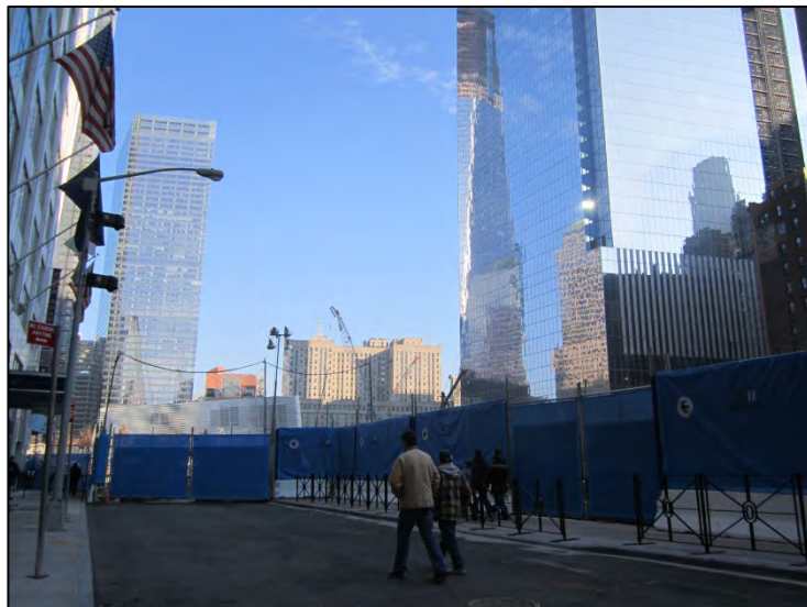
Photograph 7. On-site portion of Washington Street north of Albany Street, view north.
