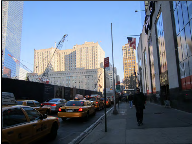
Photograph 1. On-site portion of Church Avenue north of Cortlandt Street and the west-adjacent World Trade Center construction site, view north.
