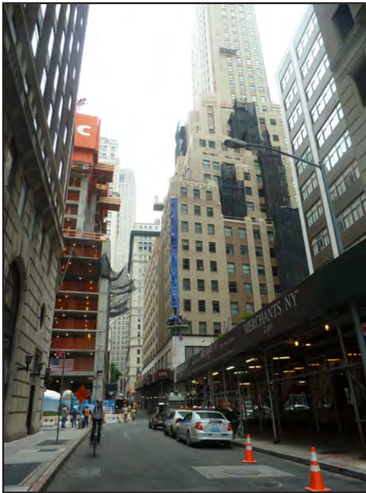
13. View east across Rector Street towards the intersection with Washington Street.
