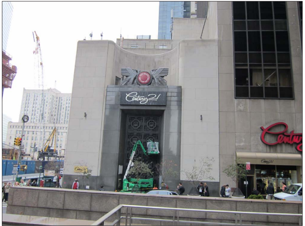
View north to the former East River Savings Bank building at 26 Cortlandt Street 7
