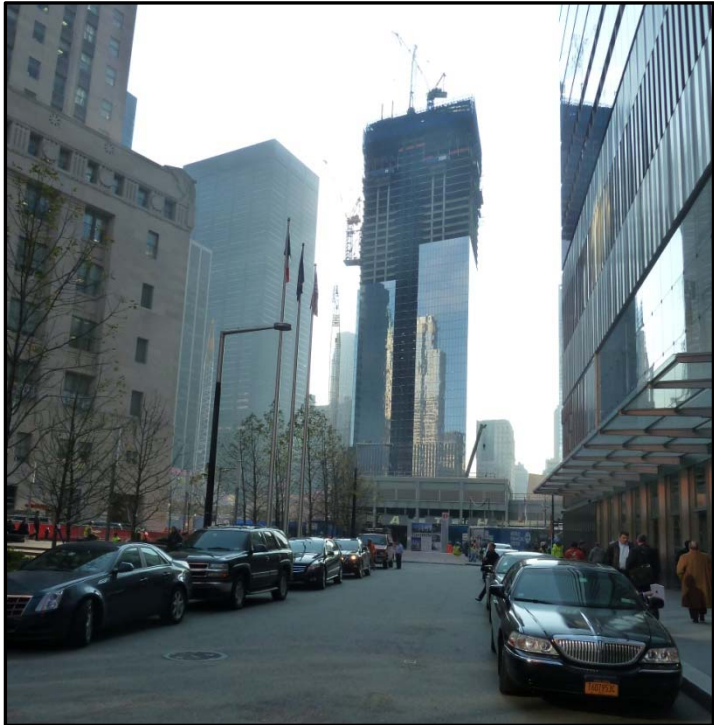
2. View of 4 World Trade Center from the north.
