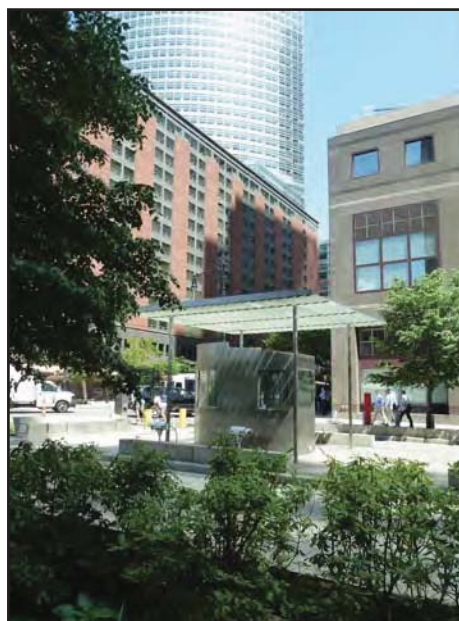
20. Guard booth at the intersection of Vesey Street and North End Avenue.
