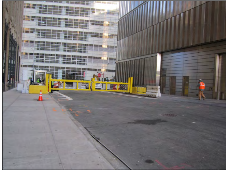
Photograph 9. On-site portion of Washington Avenue north of Vesey Street, view north.
