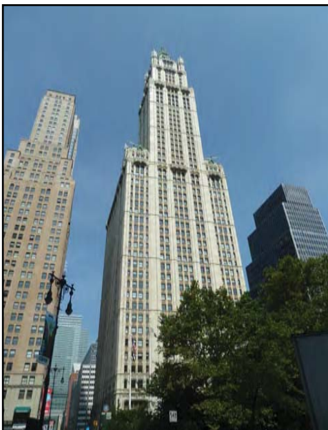
7. East facade of the Woolworth Building as seen from City Hall Park.
