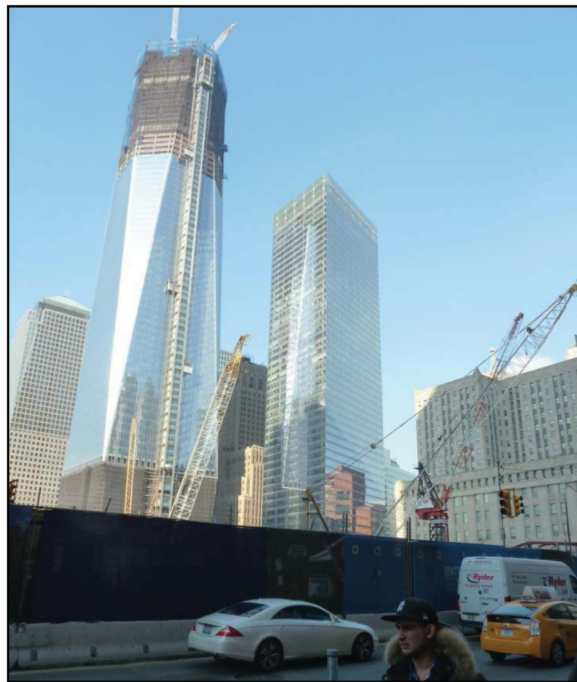
4. View west across Church Street to 1 World Trade Center.
