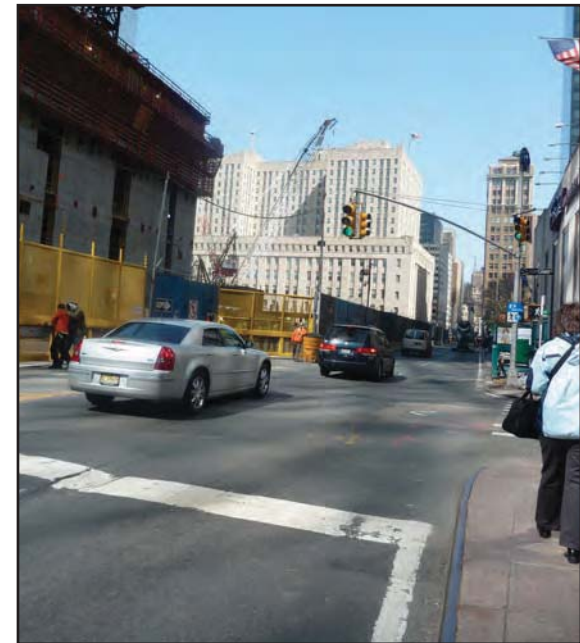
12. Existing view north along Church Street from Cortlandt Street.
