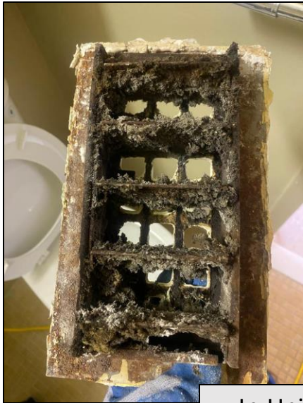
In-Unit Vent Cleaning
