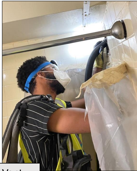
In-Unit Vent Cleaning
