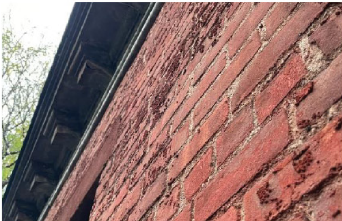
Flaking Paint Residue
