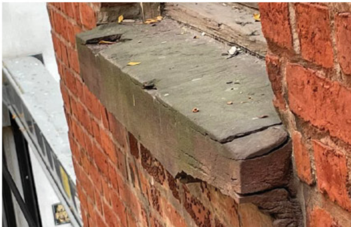
Stone Sill Deterioration
