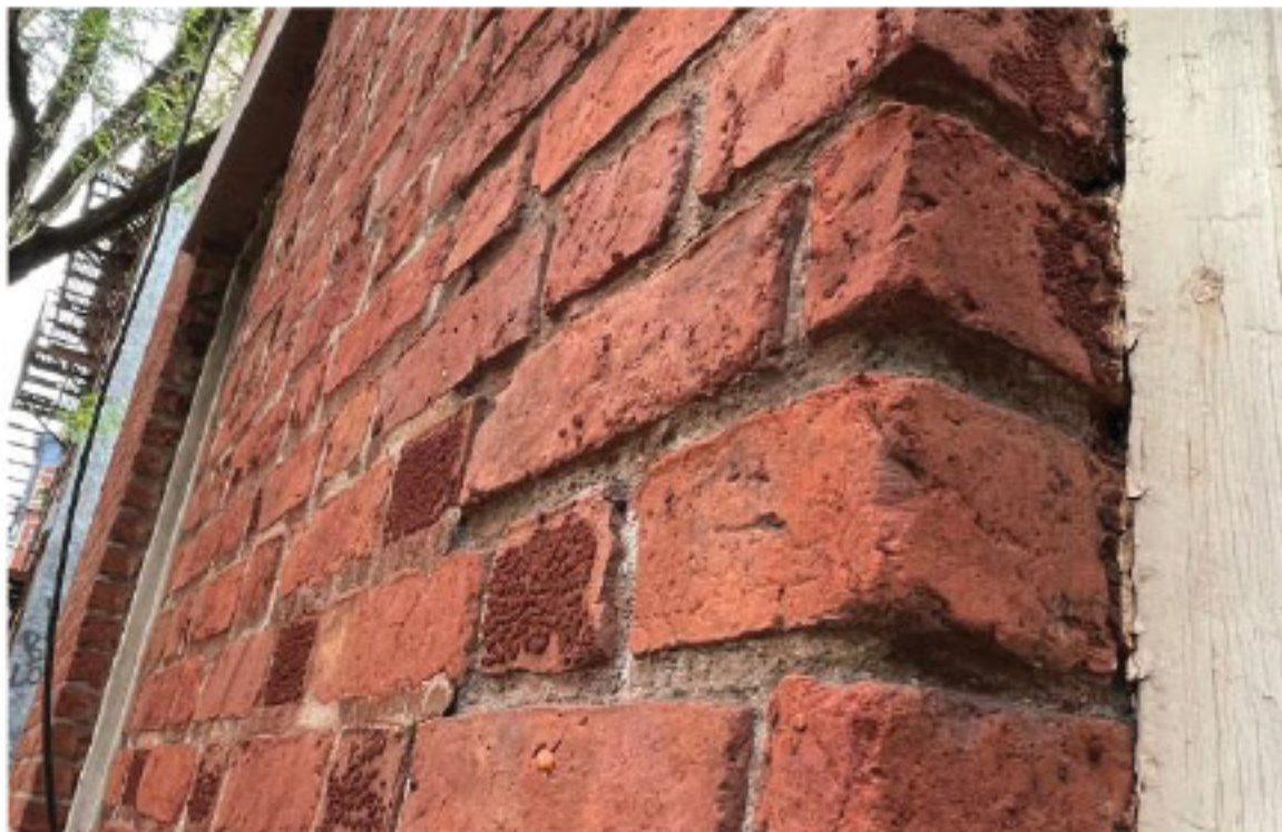
Mortar Erosion
