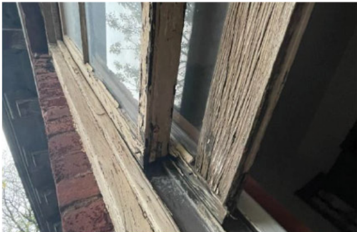
Severe Window Frame Deterioration
