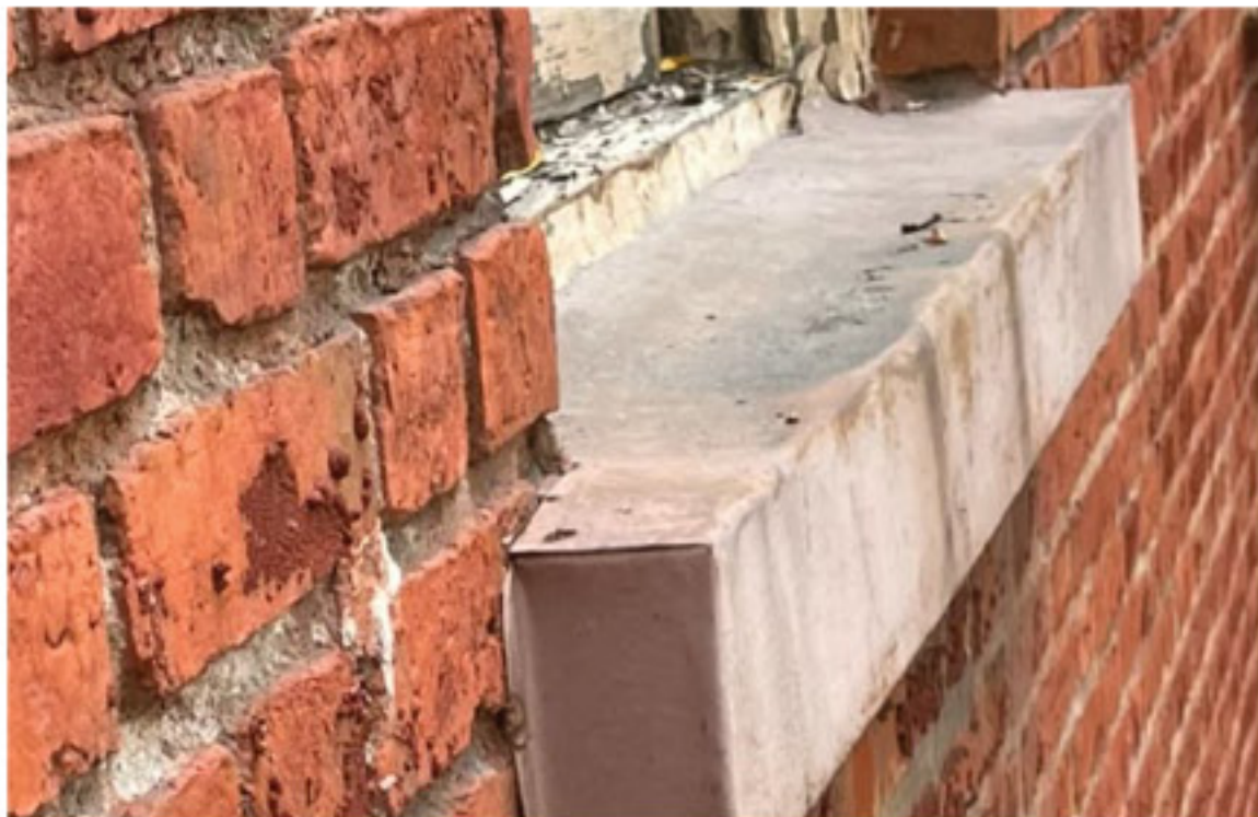
Sill Covered in Break Metal
