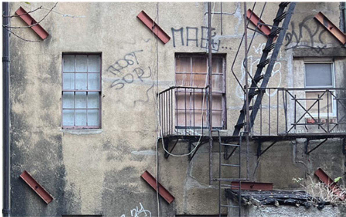
Exposed Structural Tie-Backs Installed in 2009 to help stabilize the building and prevent further separation of the facade
