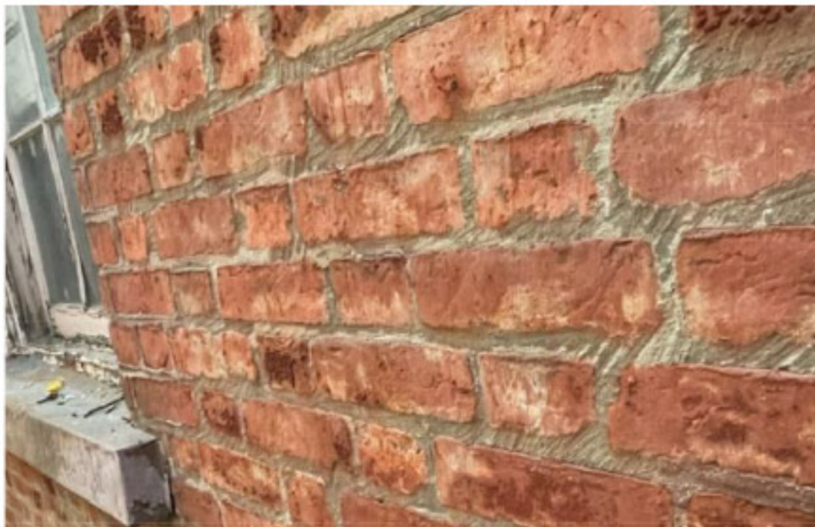
Mechanically Scraped Bricks
