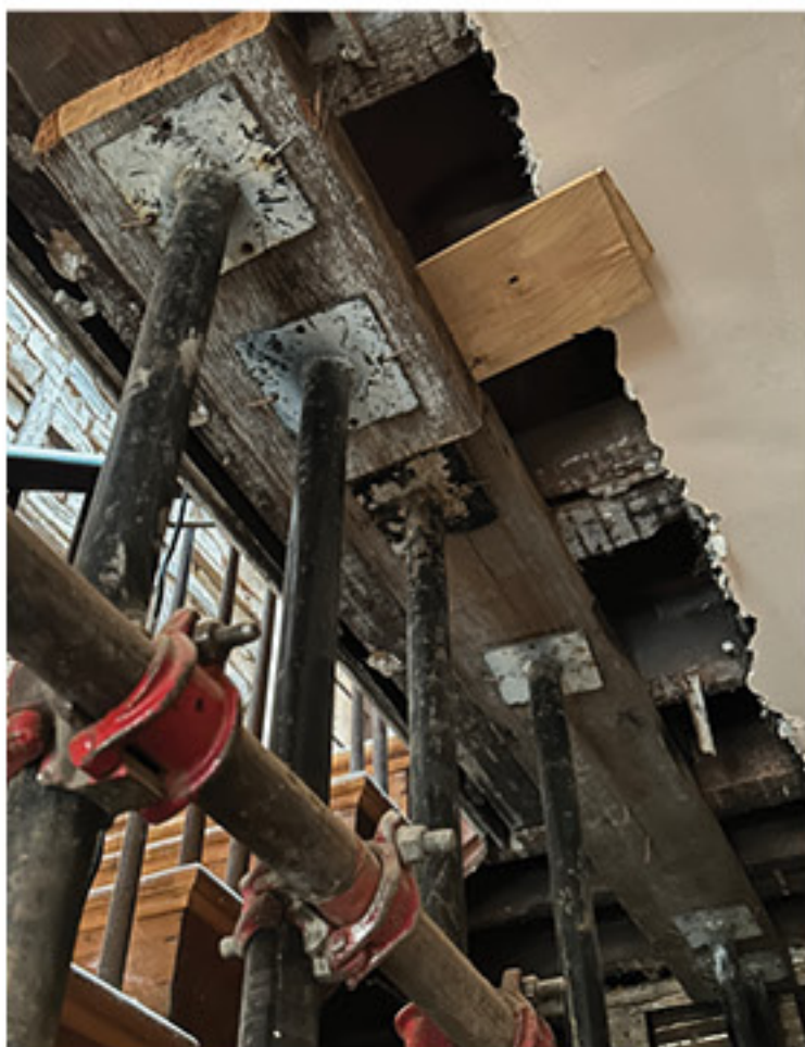
Structural shoring, installed in 2009 to prevent building collapse
