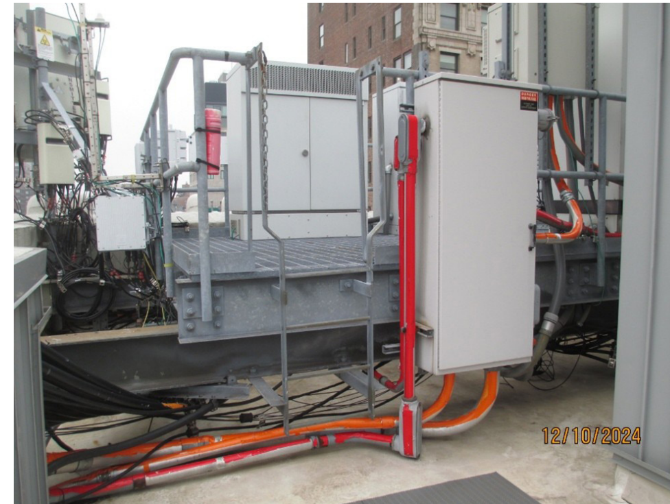
East parapet roof dunnage
