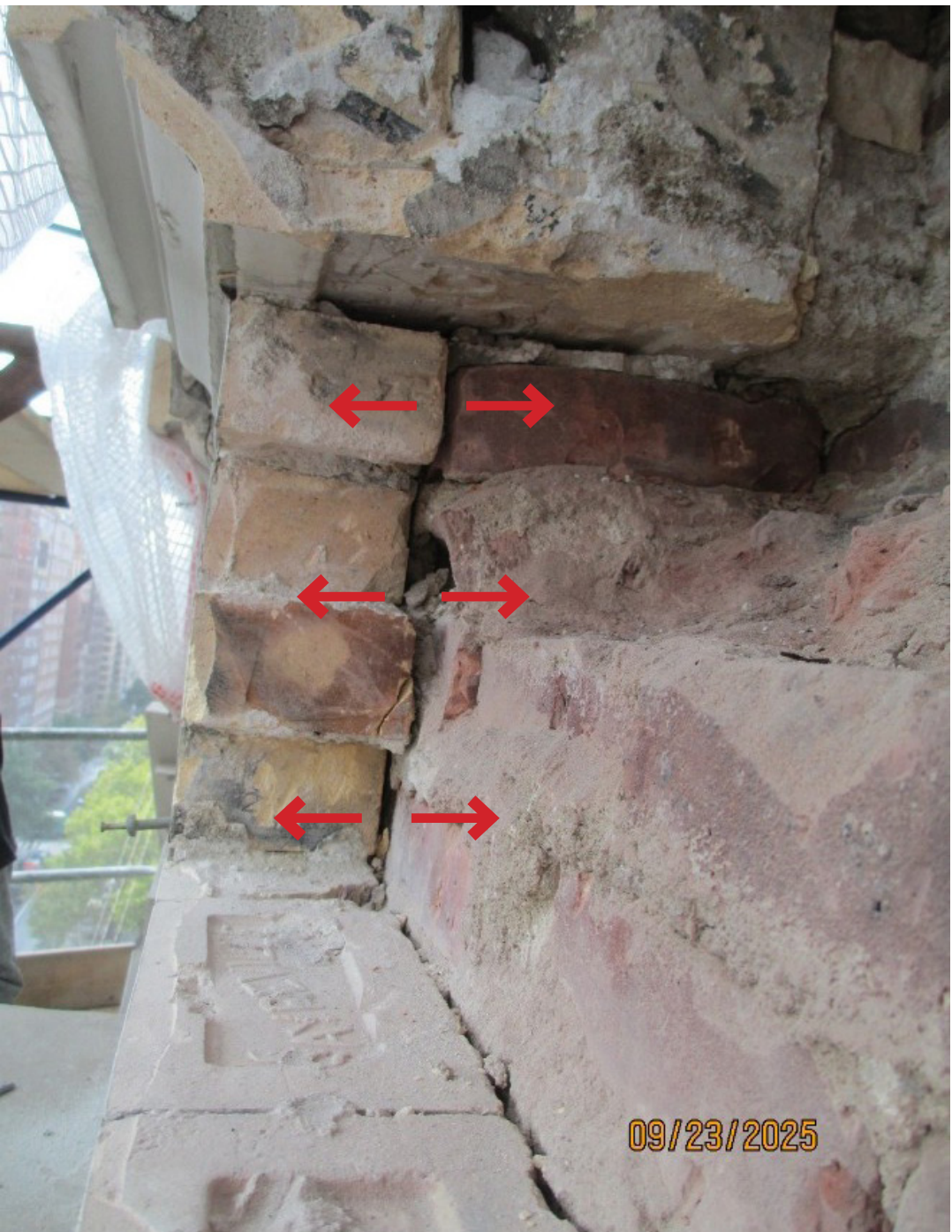
Separation between face brick and back-up brick masonry back up wall due to lack of header course
