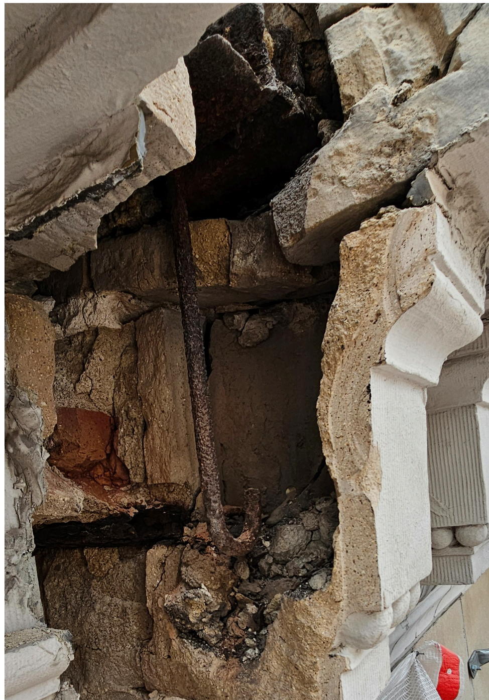
Deterioration of steel anchor embedments
