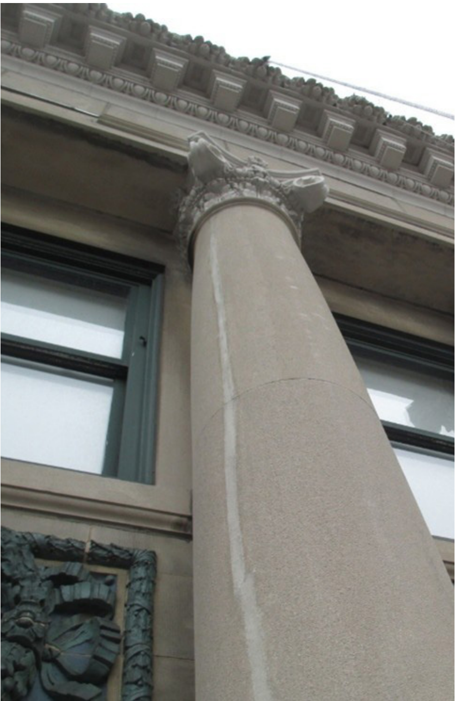
Continuous vertical cracking at limestone due to compression forces
