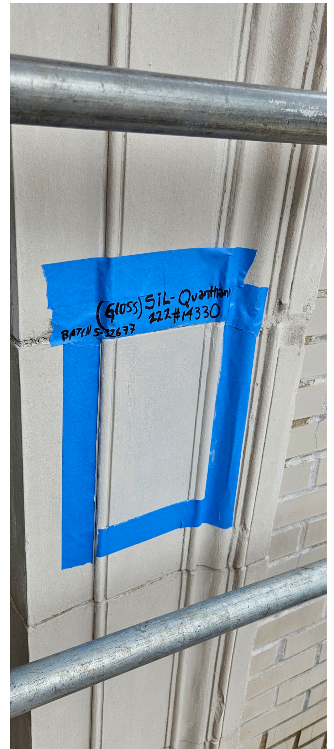
Staff Level Restoration Custom coating to match existing Edison Coatings Inc. Aquathan breathable coating
