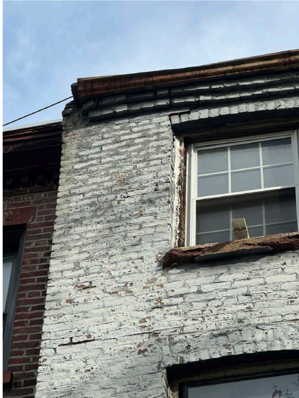
The corbeled cornice is deforming outwards as is the upper portion of wall.
