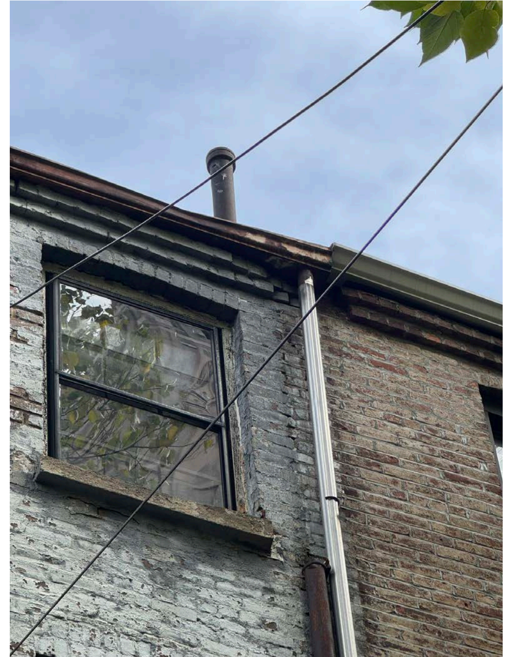
Signs of mortar fretting are present at multiple locations across the rear facade.
