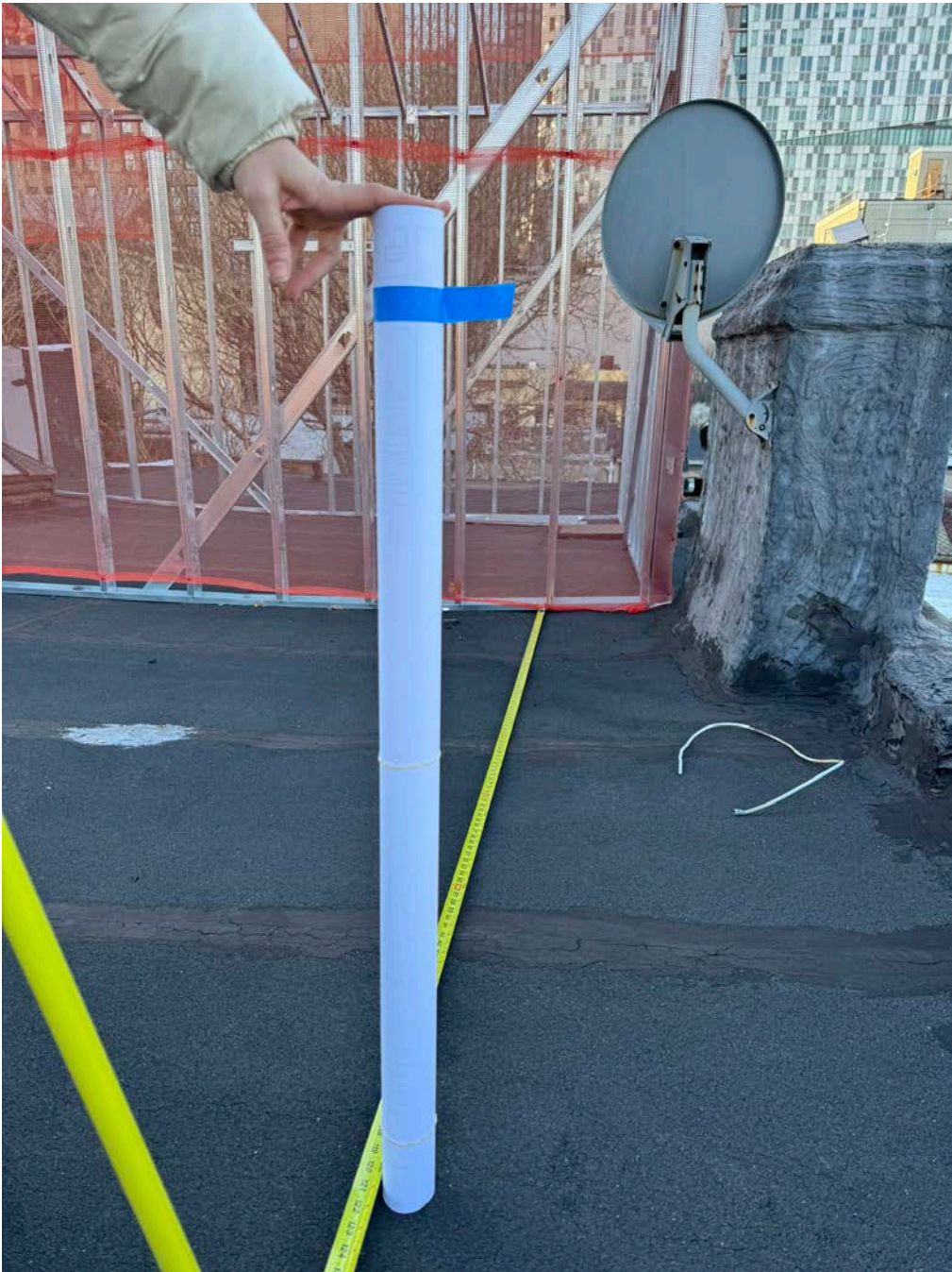
Top of blue tape indicates top of 42” railing measured from finished surface of exterior terrace.
