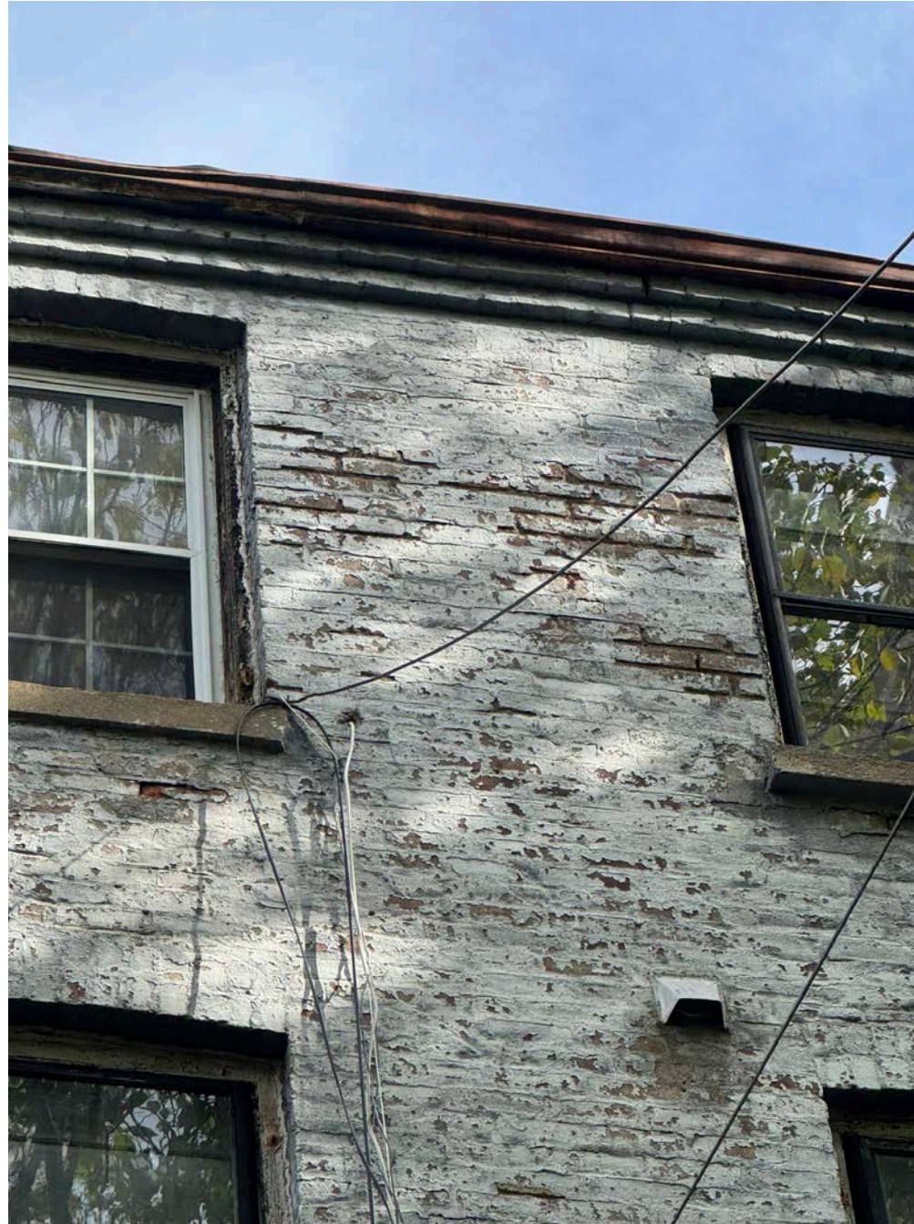
Brick spalling is present, likely due to trapped moisture behind painted finish.
