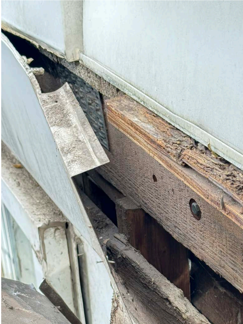
Connections are non-historic metal fasteners (bolts and gang nails). Siding is degrading vinyl.
