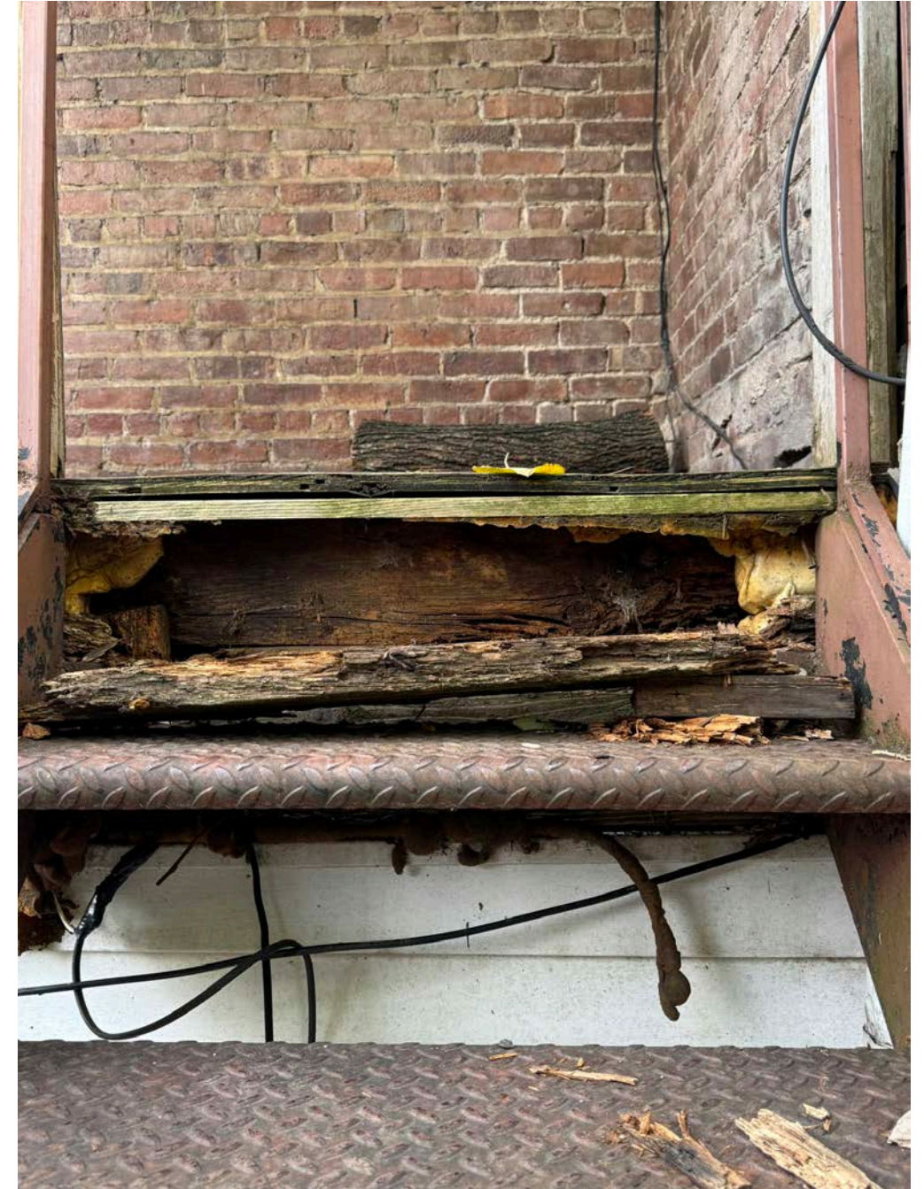
Structure is rotting out from within due to apparent water damage and poses unsafe conditions.
