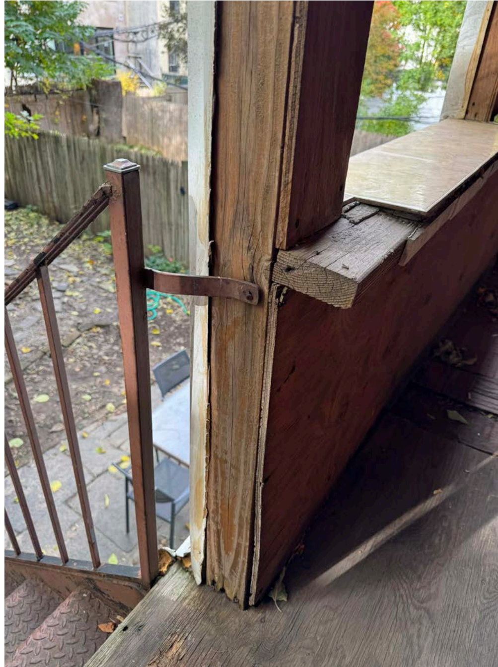
Structural posts are assembly of non-historic dimensional lumber and sheet material.
