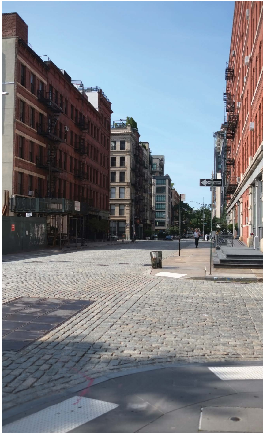
An intersection with tinted concrete paving, granite curbs and detectable warning units next to Belgian block streets.
