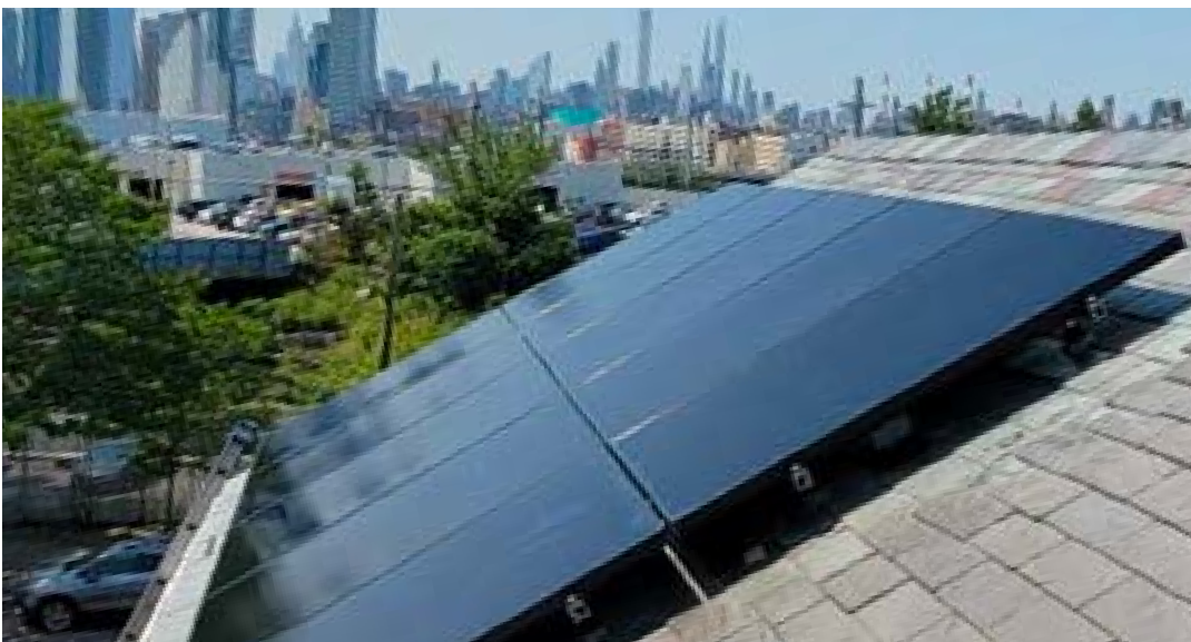
"Black-on-black" solar panels installed on slate roofing at a rear-facing sloped roof.
