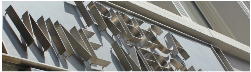
Pin-mounted lettering on a sign panel.
