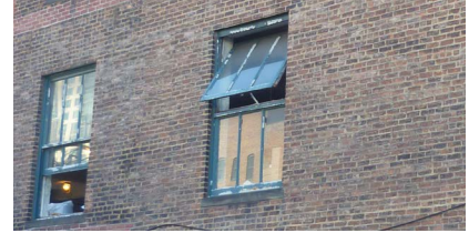
The operation of a pivot window may be changed to hinged.
