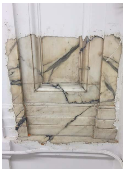
Coating removal without damaging the historic material
