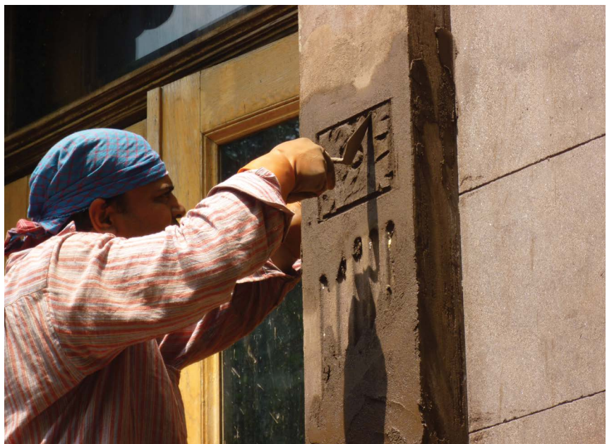
Resurfacing ornament with cementitious brownstone-tinted stucco to replicate historic details.
