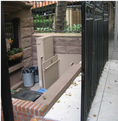
A metal platform lift installed within an areaway, finished to match the surrounding brownstone and screened by ironwork.
