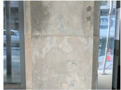
Coating would be appropriate in this case where cleaning revealed staining and previous repairs.
