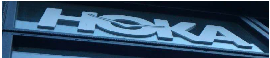
Dimensional letters that project from the exterior of the glass installed on the transom glass of a storefront.
