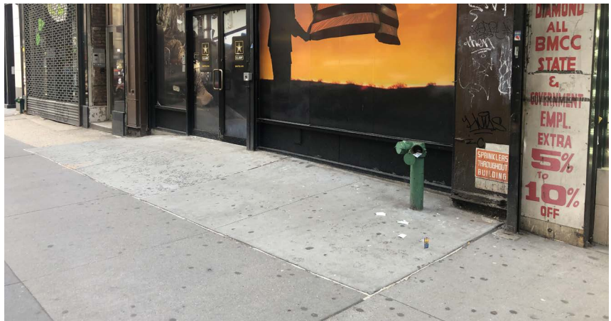
This concrete sidewalk has been sloped towards the storefront to make it accessible.
