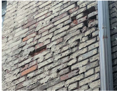
The coating used on the bricks resulted in severe deterioration of the brickwork.
