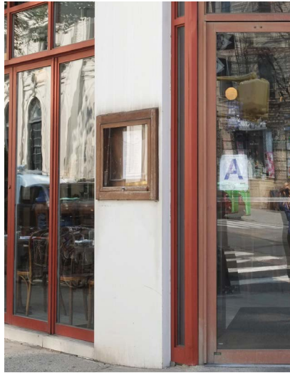
A menu box installed at areas of plain masonry at a corner storefront.
