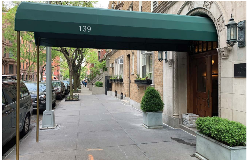
This sidewalk canopy has a design consistent with a typical historic canopy. The installation fits within the opening and does not obscure or damage significant features.
