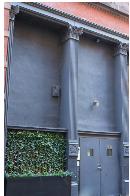
This service entrance has been infilled with a planter. Staff can issue permits approving the removal of such non-historic infill and installing new infill or a storefront in some cases.
