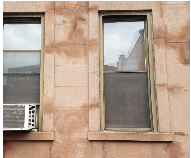
Example of inappropriate coating. Repair mortars and patching compounds should be tinted to match the original material, not the coated and/or stained materials.
