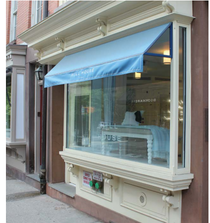
A fixed storefront awning installed at the top of the projecting display window.
