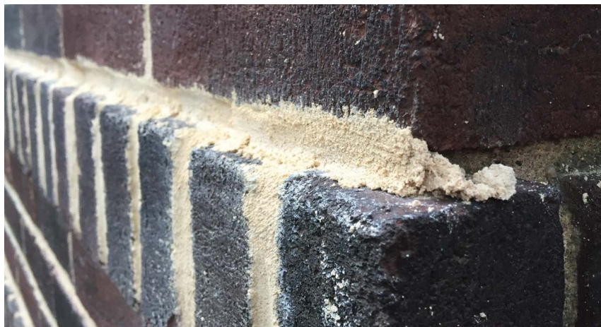
Example of inappropriate mortar joint repointing. Note how the new mortar has been layered on top of the old mortar, overlapping the brick faces and covering the joints rather than filling them.
