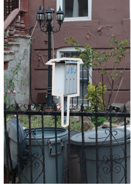
Mailboxes can also be installed on a freestanding post in an areaway.
