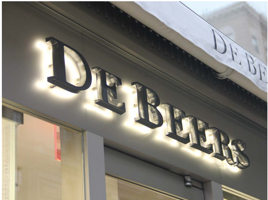
Halo-lit, pin-mounted lettering at a signband.
