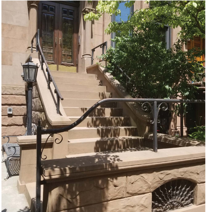
A simple metal railing has been installed on the top of this masonry stoop for safety.
