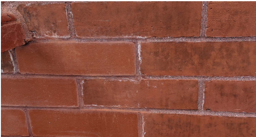
New brick that matches the historic brick in terms of size, dimensions, and finish.
