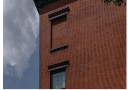
A filled-in window opening at a secondary facade.
