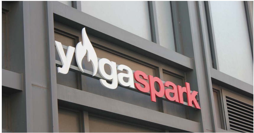
Lettering mounted on a metal channel within a transom.
