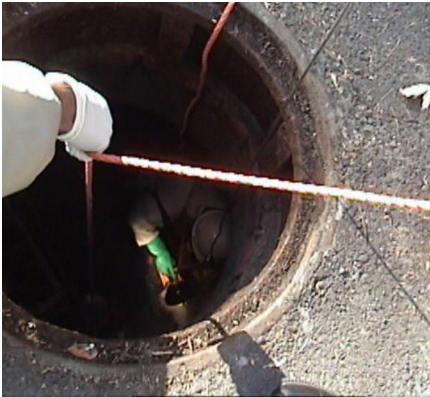
DEP staff begins sewer investigation
