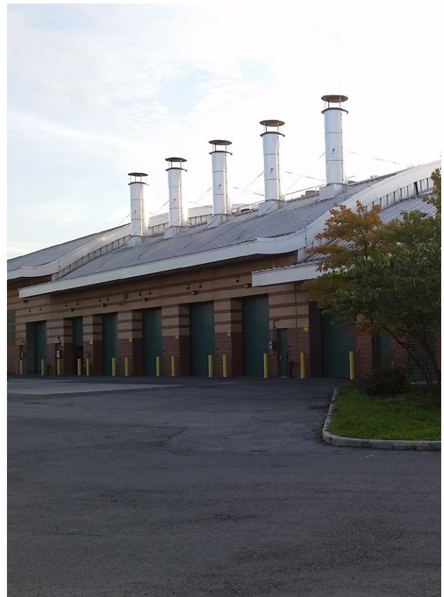
Paerdegat Basin CSO facility
