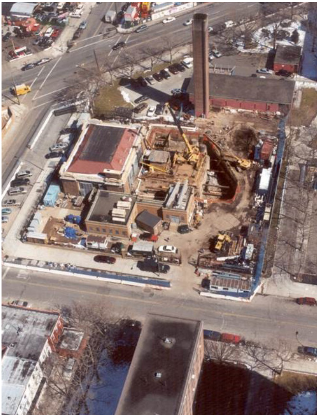
Construction at Avenue V pump station
