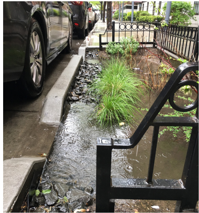
Rain garden construction in Flushing, Queens
