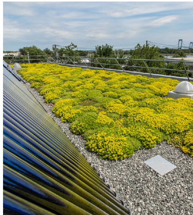
Green Roof at Zerega EMS Station
