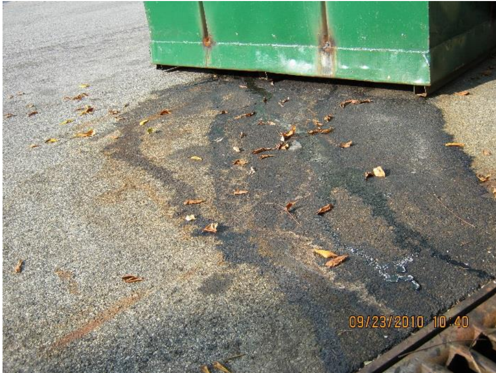
Image 1.1 Visual observation of dumpster leaking into a storm sewer (source: sustainablestormwater.org)
