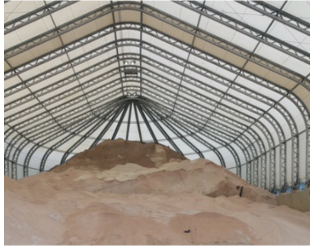
DSNY salt shed
