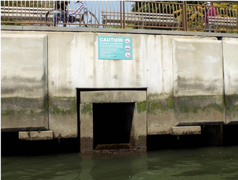
NCM-042 - Outfall in Good condition
