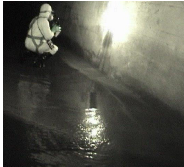
DEP staff conducts in-sewer investigation
