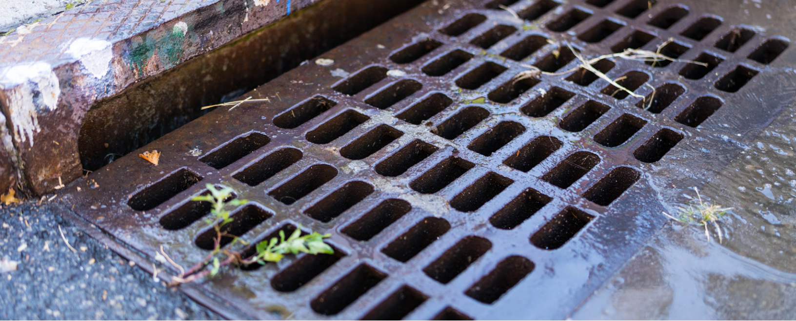
Discharge entering a storm drain.
