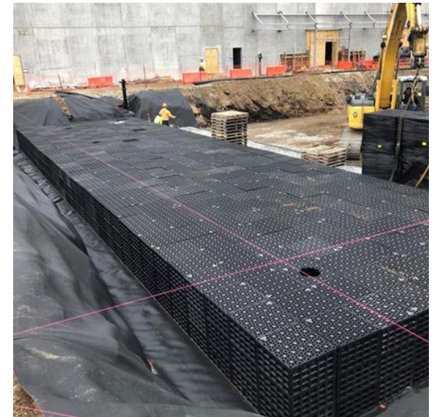
Proposed subsurface storage system
