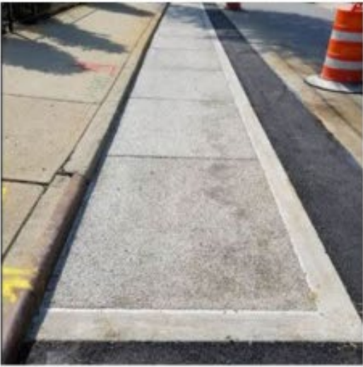
Porous Pavement bike lanes and parking lanes
